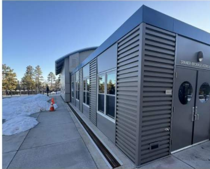
FLAT ROOFED STATIONARY PORTION Closed position.
